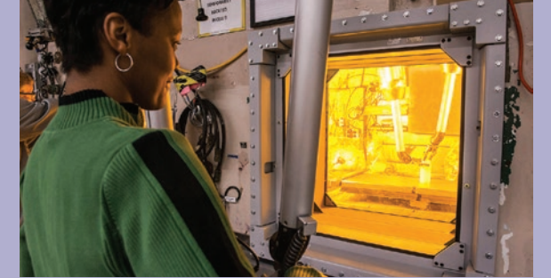
Shielded Cells used for fuel dissolution and first cycle solvent extraction.
