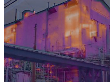
Thermal image of the Honeywell Metropolis Uranium conversion facility during restart activities.
