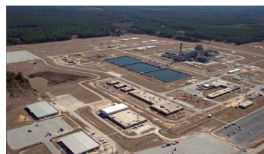
Decommissioned Reactor Range
