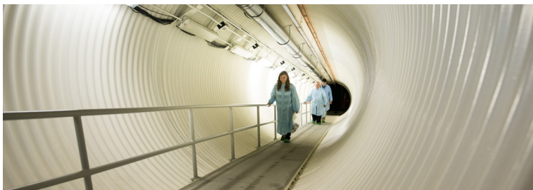
Underground Counting Facility
