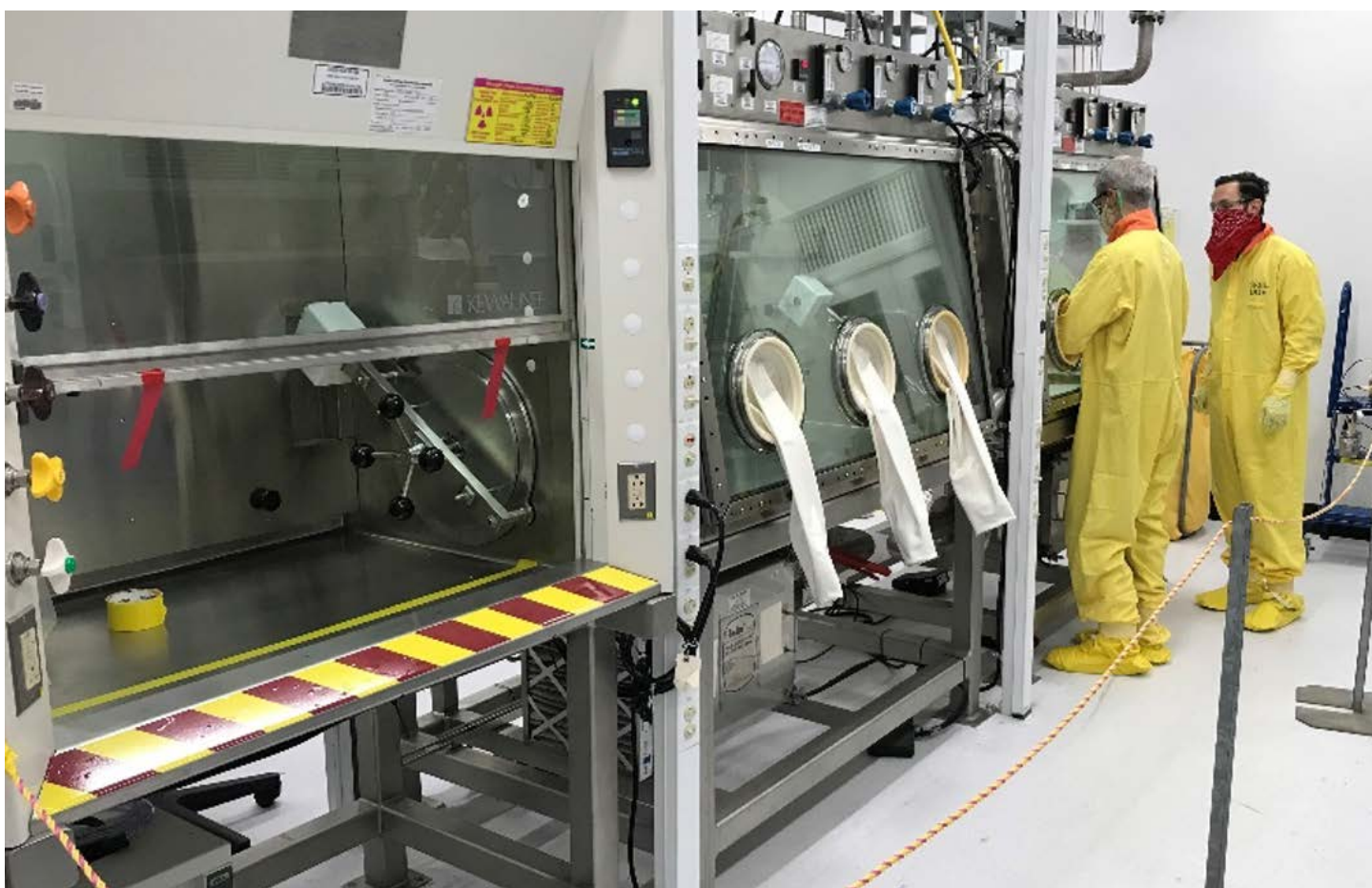
Figure 4: LDRD researchers study enriched uranium materials inside a radiological glovebox within SRNL's Category II nuclear facility.
