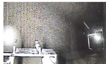
Figure 2. Human denied H-CAEX tunnel interior view
